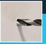
Drill a 10mm hole in the substrate.
